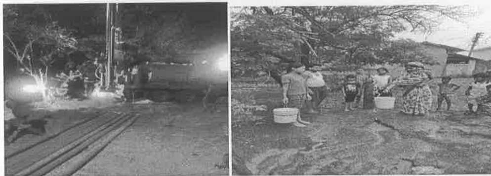
Photo 2: Drilling of bore well and installation of the submersible pump at village Baispali.
