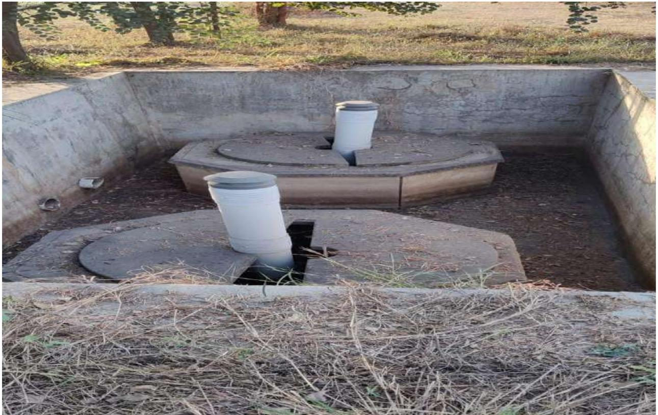
**Fig 7.1: Rain water Harvesting in the plant premises**
