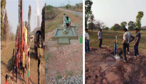
\* Drilling of bore well & Installation of Submersible pump & Hand pump at Labour colony, Badadarha, CHC and near weigh bridge at Basanpali respectively
